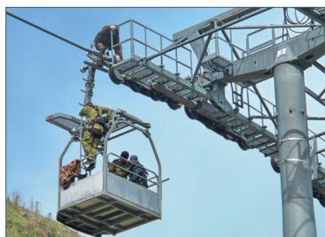
Cable car construction
