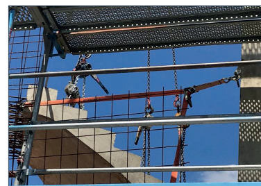
Positioning of loads
